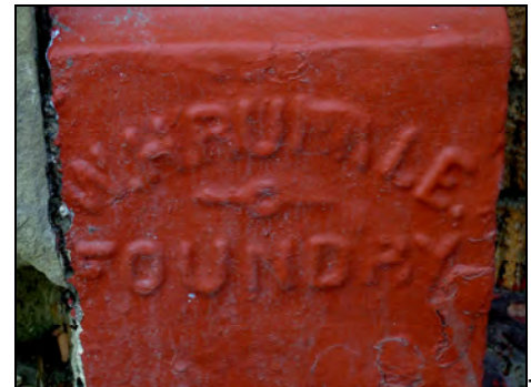
Runkle column, 129-31 West Main St.
