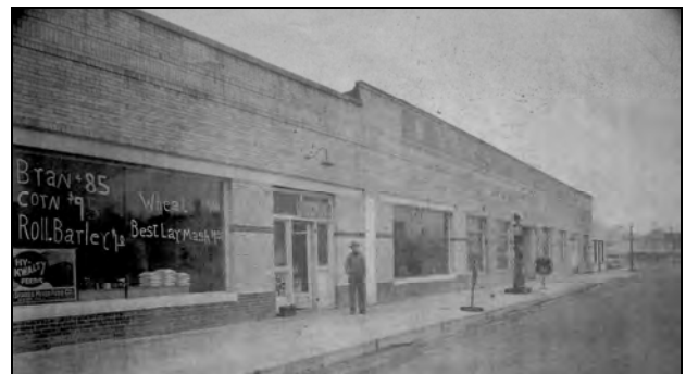
Figure 16. A number of one-story brick buildings, mostly housing automotive-related businesses, were built along W. Front Street in the 1920s, including (from left to right) 119, 121-23, and 129 West Front Street. SOURCE: Price Pioneer Museum, photograph collection, Florence, Colorado.
